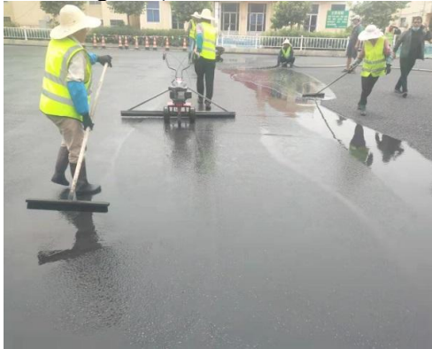
1) Cement-based Grout is Scraped
