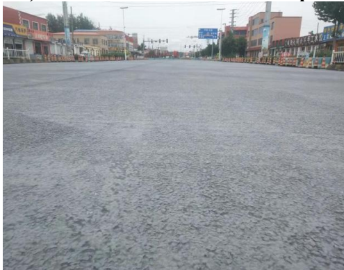
2) The Pavement after Grouting is Completed
