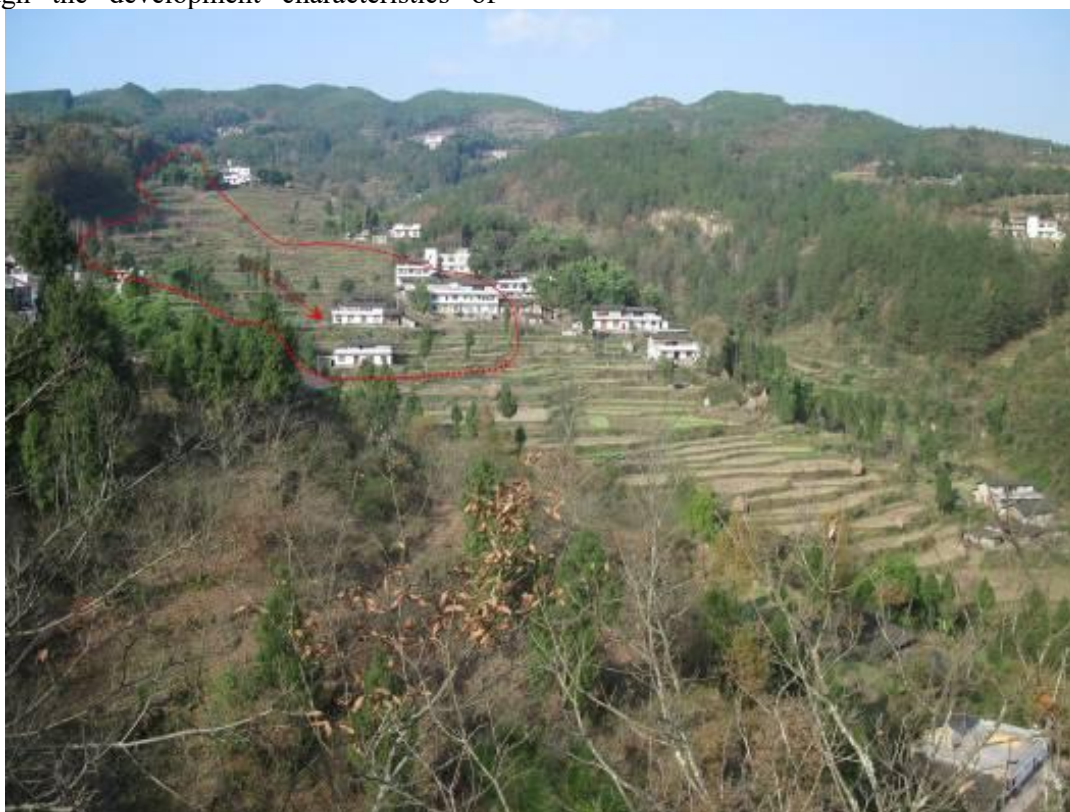
Figure 1. Overall View of Landslide
