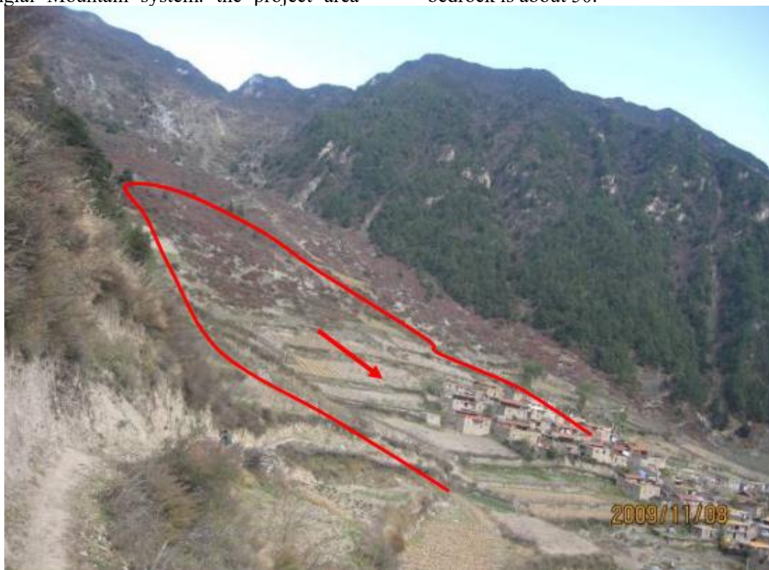
Figure 1. Panorama of Mixed Ditch Landslide
