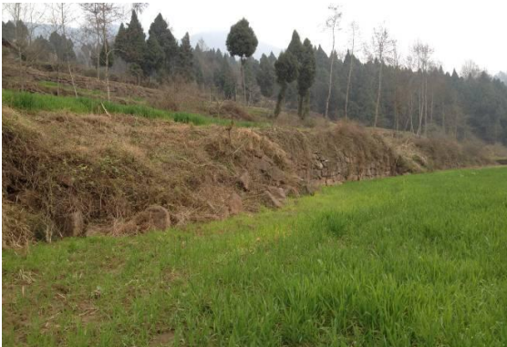
Figure 1. Collapse of the Front Edge of the Landslide and Tilting of Trees
