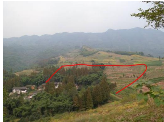
Figure 1. Overall View of Landslide
