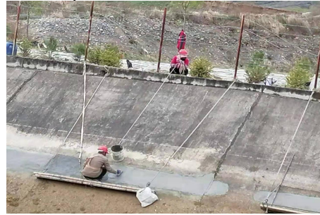
Figure 1. Construction-Specific Work Platform
