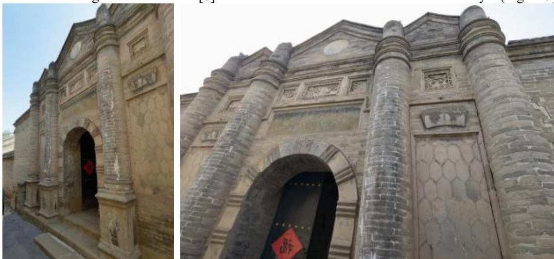
Figure 9. East-West Integration in the Mao's Compound Image Source: Photo Taken by the Authors
