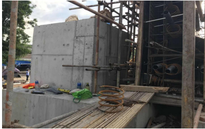
Figure 1. Construction Site of Slotted Beam
