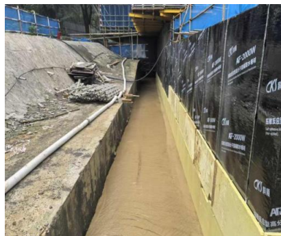
Figure 3. Fluidised Stabilised soil Backfilling Construction
