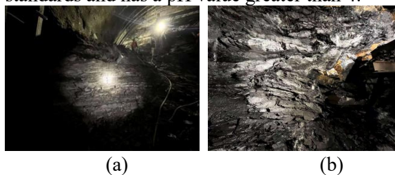
Figure 1. Mudstone Excavated During Tunnel Excavation
