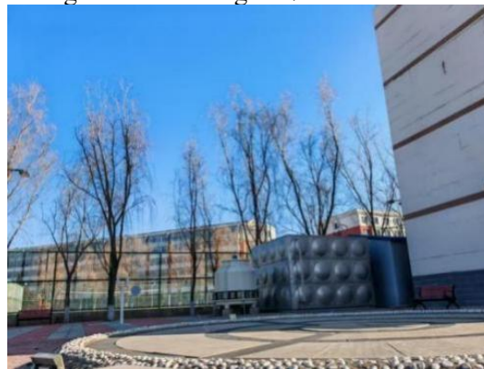
Figure 7. Fountain Installation on the West Side of the Logistics Building
